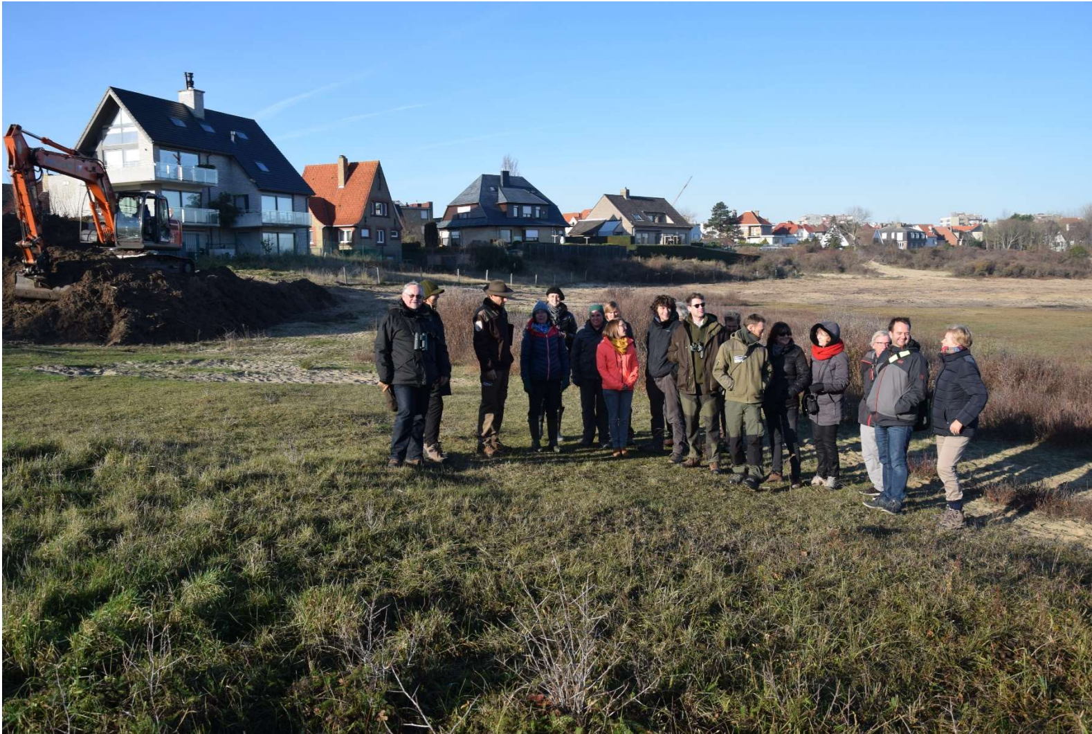
The advisory committee of LIFE+ FLANDRE visits the nearly completed works (please note the crane on the far left of the picture) in the western part of the Houtsaegerduinen on 12 December 2018
