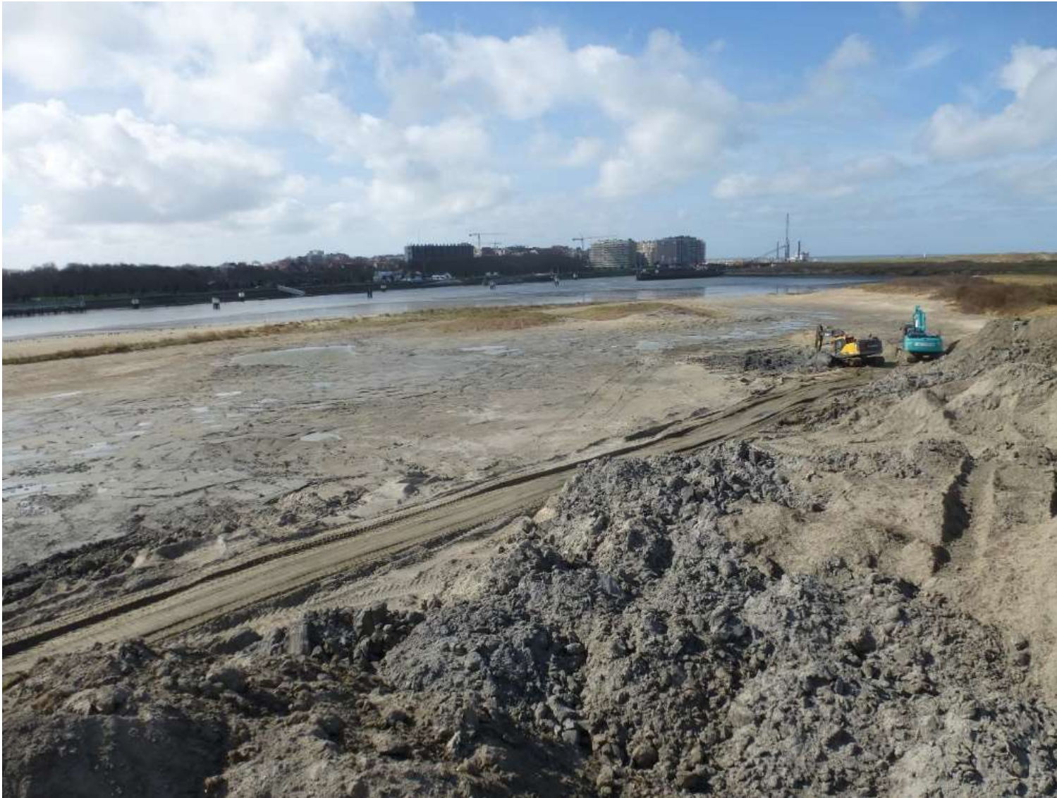
Photo: the dredging sludge dump is being excavated
