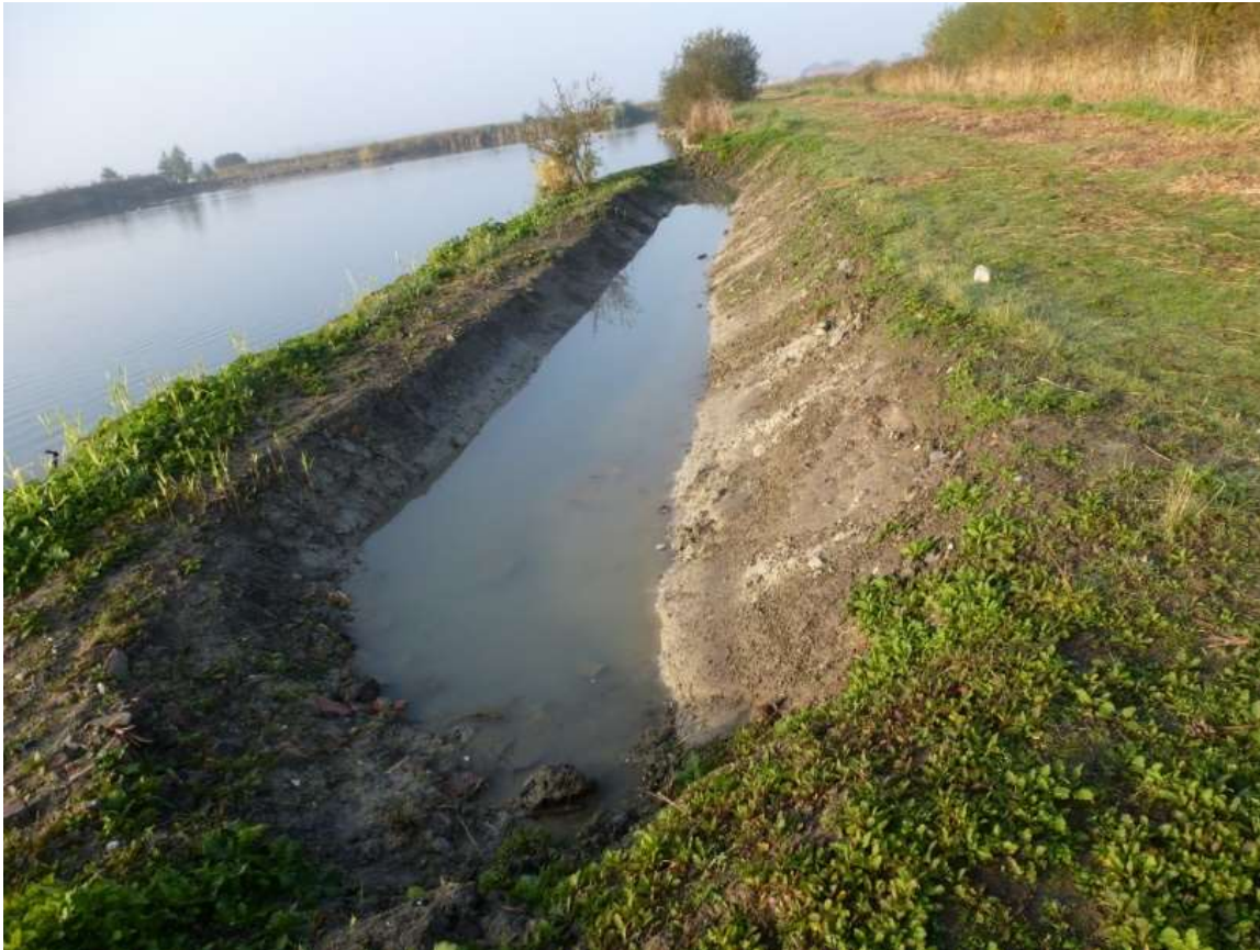
Photo: newly created shallow ditch along the banks of the pond 'Drie Vijvers' at 'Zwarten Hoek'
