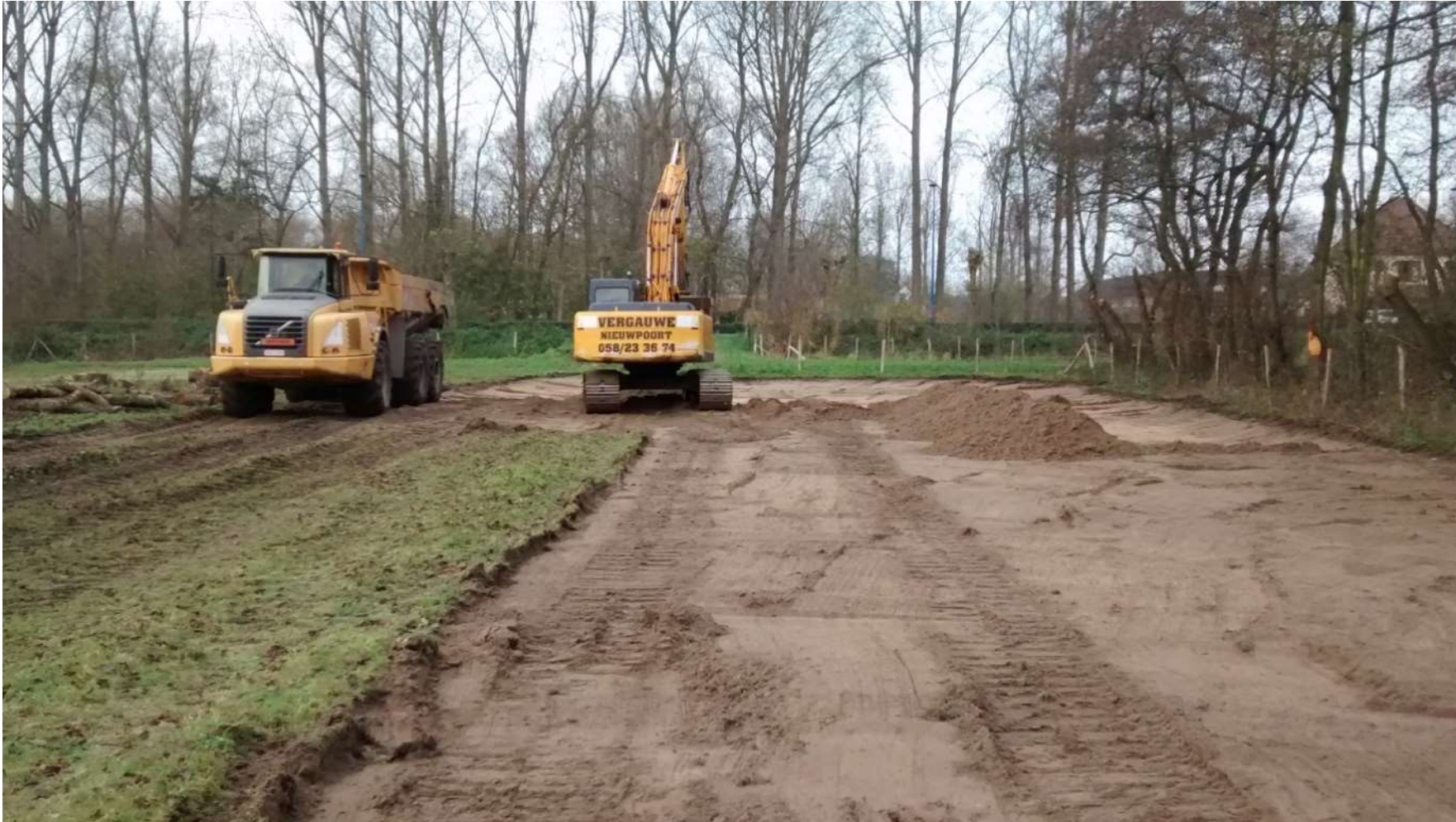
Photo: excavation of the topsoil at the 'Fluithoek'
